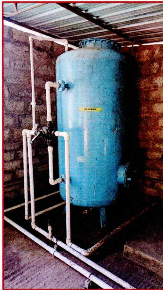
Figure 9 Dual Media Filter
