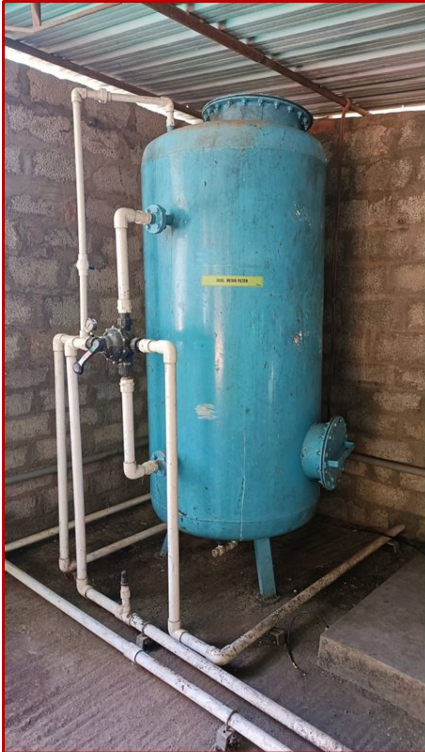
Fig. 4.8 Dual Media Filter
