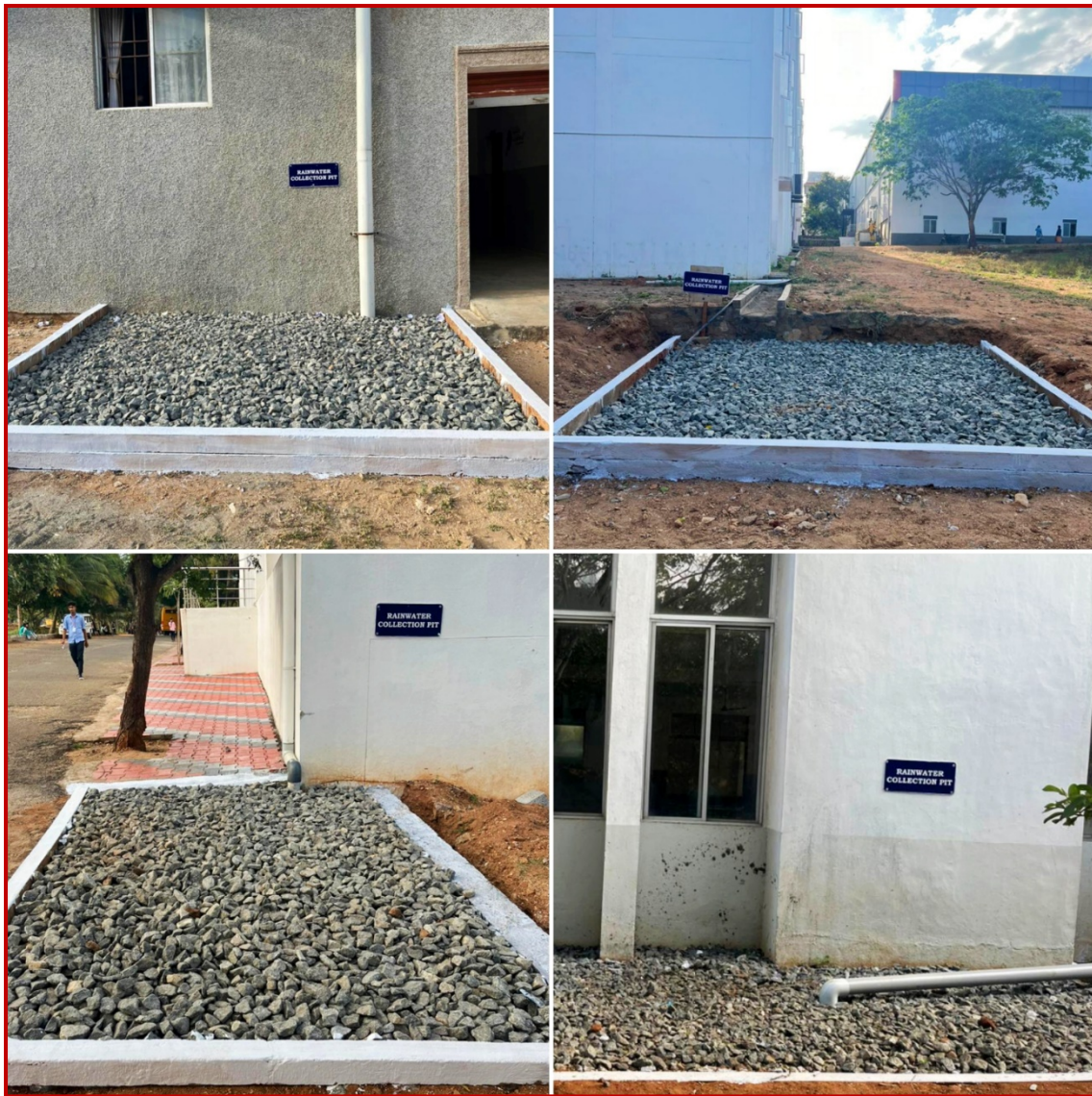
Fig. 4.2 Rainwater Harvesting Pits
